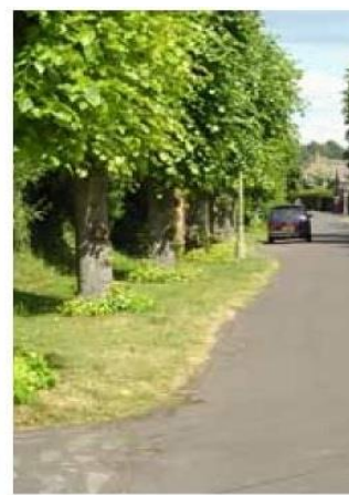
THE ROADS ON THE TOP OF THE HILL ARE UNADOPTED AND HAVE SOFT VERGES
